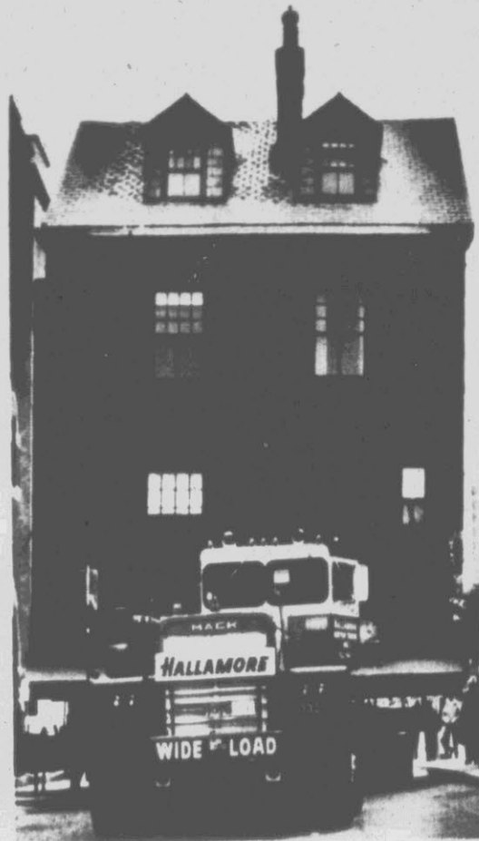
HOUSE MOVING — Truck moves a 91 year old, 300 ton brick house along Blossom Street in Boston Sunday, as it begins a journey to its new site 366 yards away. The resident physician's house belonging to Massachusetts General Hospital is being moved to make way for construction of a new medical research building. (AP Laserphoto)
