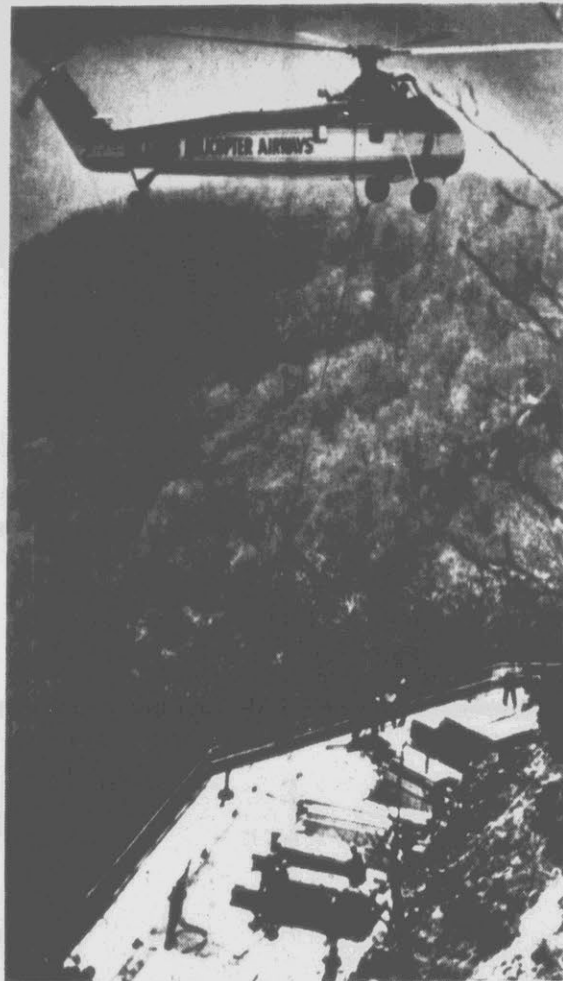
SKY LOUNGE — Chimney Rock Park's Sky Lounge atop the elevator to Chimney Rock (N.C.) burned down September 5, 1981, but the structure will soon be rebuilt as an airlift brought prefabricated sections for the new structure to the pad. The 10-hour operation began early Tuesday as St. Louis Helicopter Airways Inc. from Missouri airlifted 40-50 tons of building materials from the parking area to the lounge pad. Helicopter was the only way for the material to be brought to the cliff which is 25 feet above the parking elevator, and is serviced by an elevator. (AP Laserphoto)
