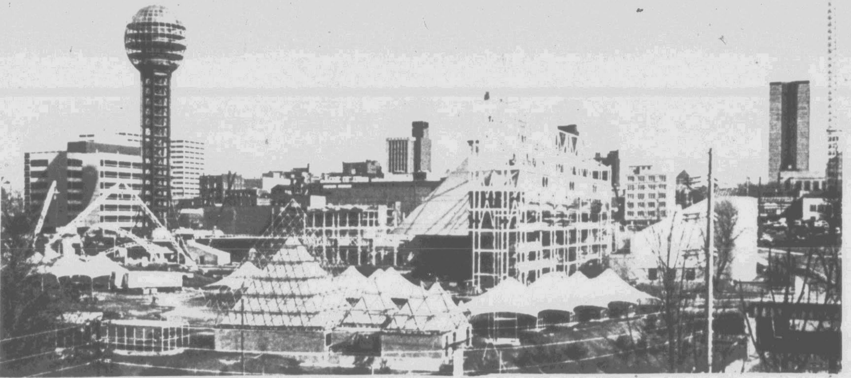
1982 WORLD'S FAIR TAKES SHAPE — The 1982 World's Fair in Knoxville, Tenn. begins to take form as the exposition's permanent buildings and dramatically shaped tension structures spring up on the Fair site. In the upper left, the Fair's theme structure, the 266-foot high Sunsphere,
