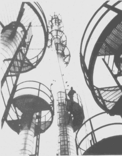
SHIPS AHOY? — This host of crows nests surrounding a fractionate tower under construction at Pennzoil Co.'s specialties refinery at Karns City, Pa. looks as though a large ship is sitting in a harbor. The units will be used to boost output of low-odor environmentally acceptable ink oils and solvents for a rapidly growing world market for newspapers and magazine users of dry printing inks. (AP Laserphoto)
