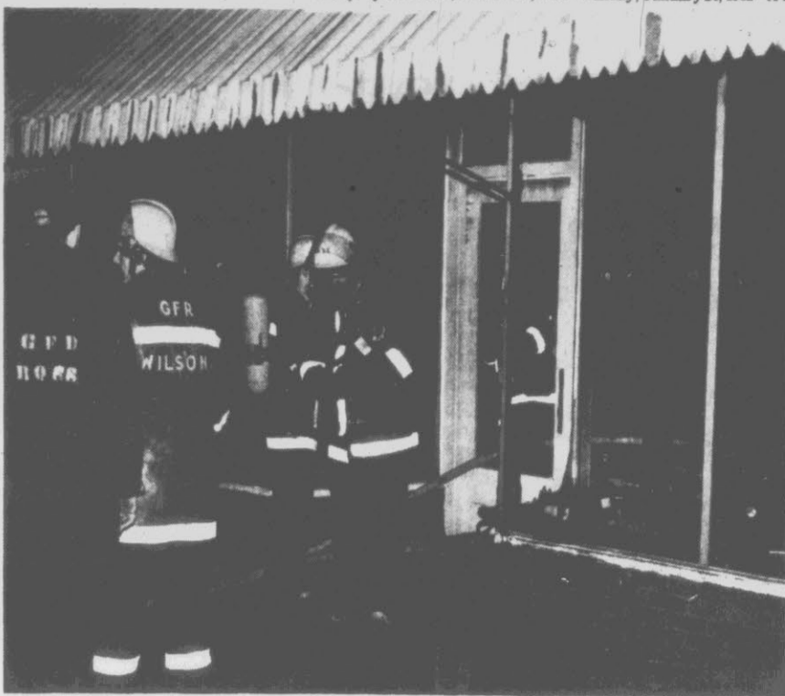
FIRE DAMAGE — The Yamaha of Greenville Dealership, 1506 N. Greene St., sustained heavy fire, smoke and water damage in a Saturday night fire. The Greenville Fire Department dispatched two trucks at 6:47 p.m. to answer the call. Firefighters arriving at the scene found the front of the building
