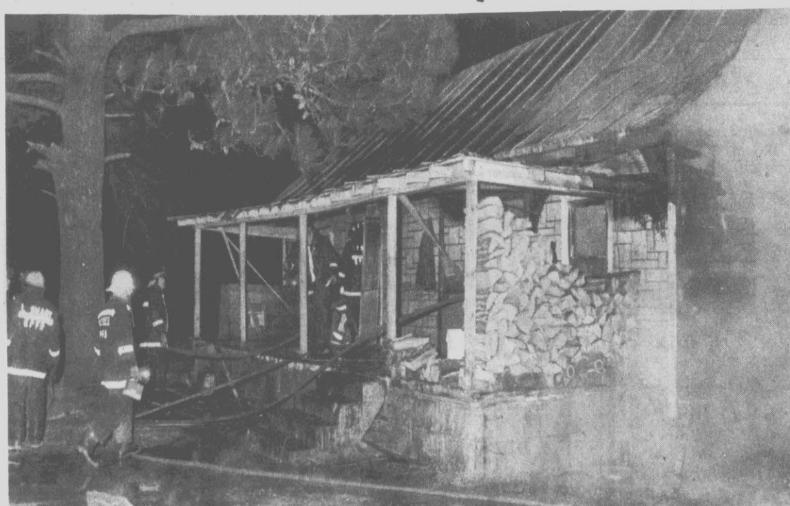
FIREMEN BRAVED LAST NIGHT'S COLD...to battle a fire at the home of Lester Mills near Black Jack. Black Jack was assisted by both Eastern Pines and Winterville. (Reflector Photo By Tommy Forrest)
