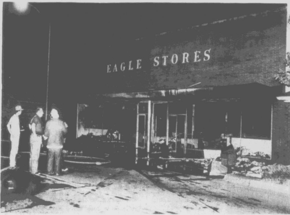
DOWNTOWN FIRE — Firefighters survey the damage to the Eagle Store on Main Street in downtown Williamston last night. Fire units from Williamston, Bear Grass, Griffins Township and Jamesville fought the 6:31 blaze, which "pretty well caused a total loss of the contents, if not the structure," according to Williamston Fire Chief Tommy Price. Damage
