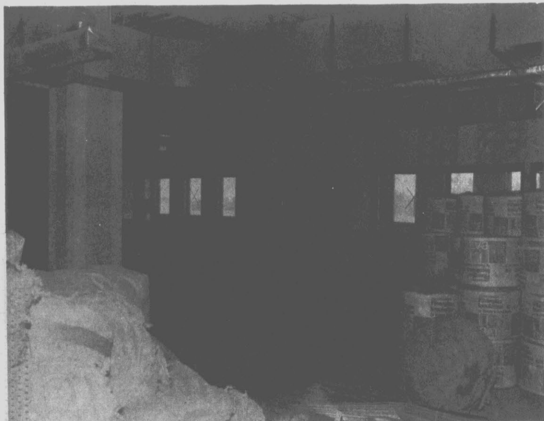
LIBRARY CONSTRUCTION — Insulation and building materials stand idle, awaiting the time they will be used, on
