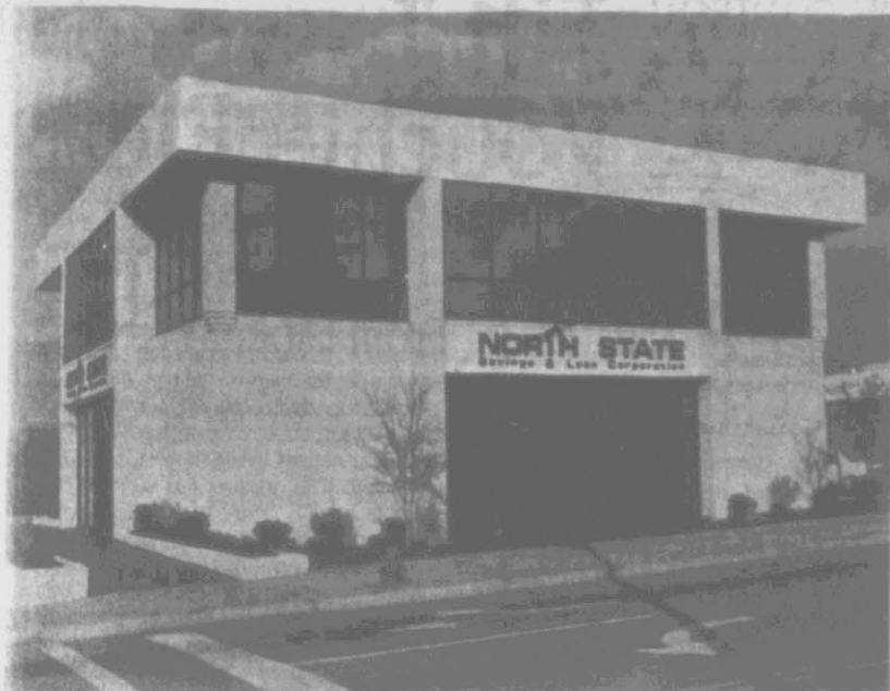
NEW FACILITY — of North State Savings & Loan Corp. at the corner of Second and Washington Streets
