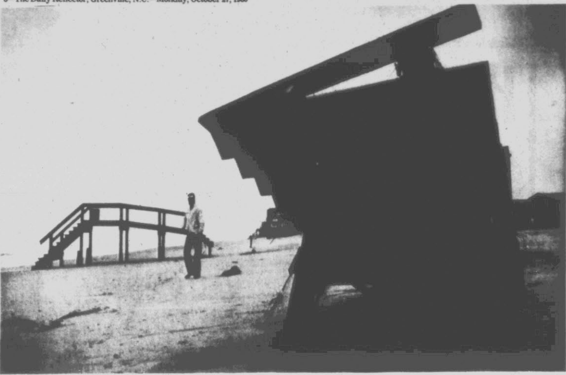
EROSION DAMAGE — Wesley Wood, of Thomasville, N.C., surveys erosion damage on the South end of Topsail Beach after last week's high tides and winds combined causing heavy
