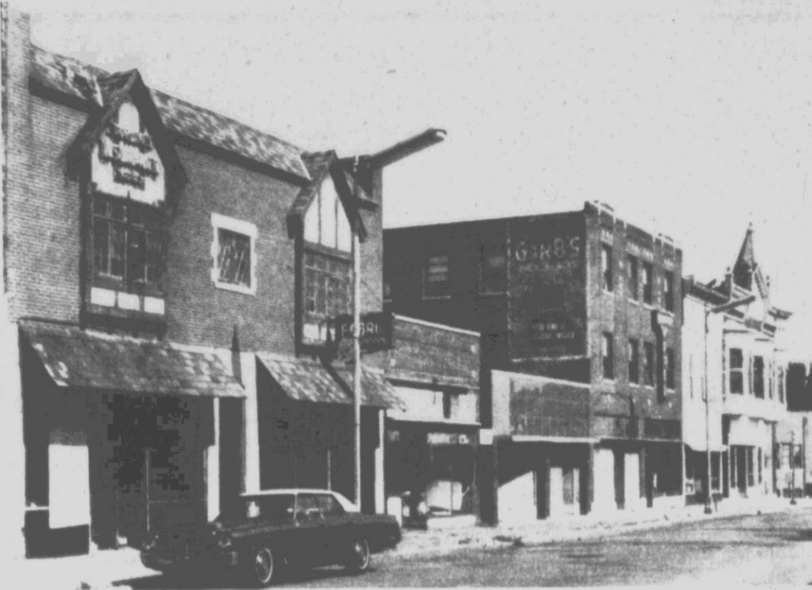
BARE BLOCK — Row of buildings in downtown Benton Harbor is vacant except for transient hotel and soup kitchen. The photo, taken earlier this summer, is typical of entire downtown area. (AP Laserphoto)
