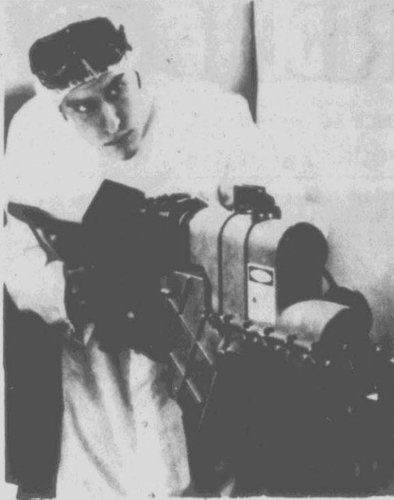
TARGET DESIGNATOR — A technician, Dennis Daniel, attaches a TV camera to the eyepiece of a Laser Target Designator at Hughes Aircraft's Culver City (Calif.) plant. The LTD will enable ground troops to pinpoint targets for laser-homing weapons or mark them for the delivery of conventional weapons. The camera is part of a system that automatically tests laser performance. (AP Laserphoto)
