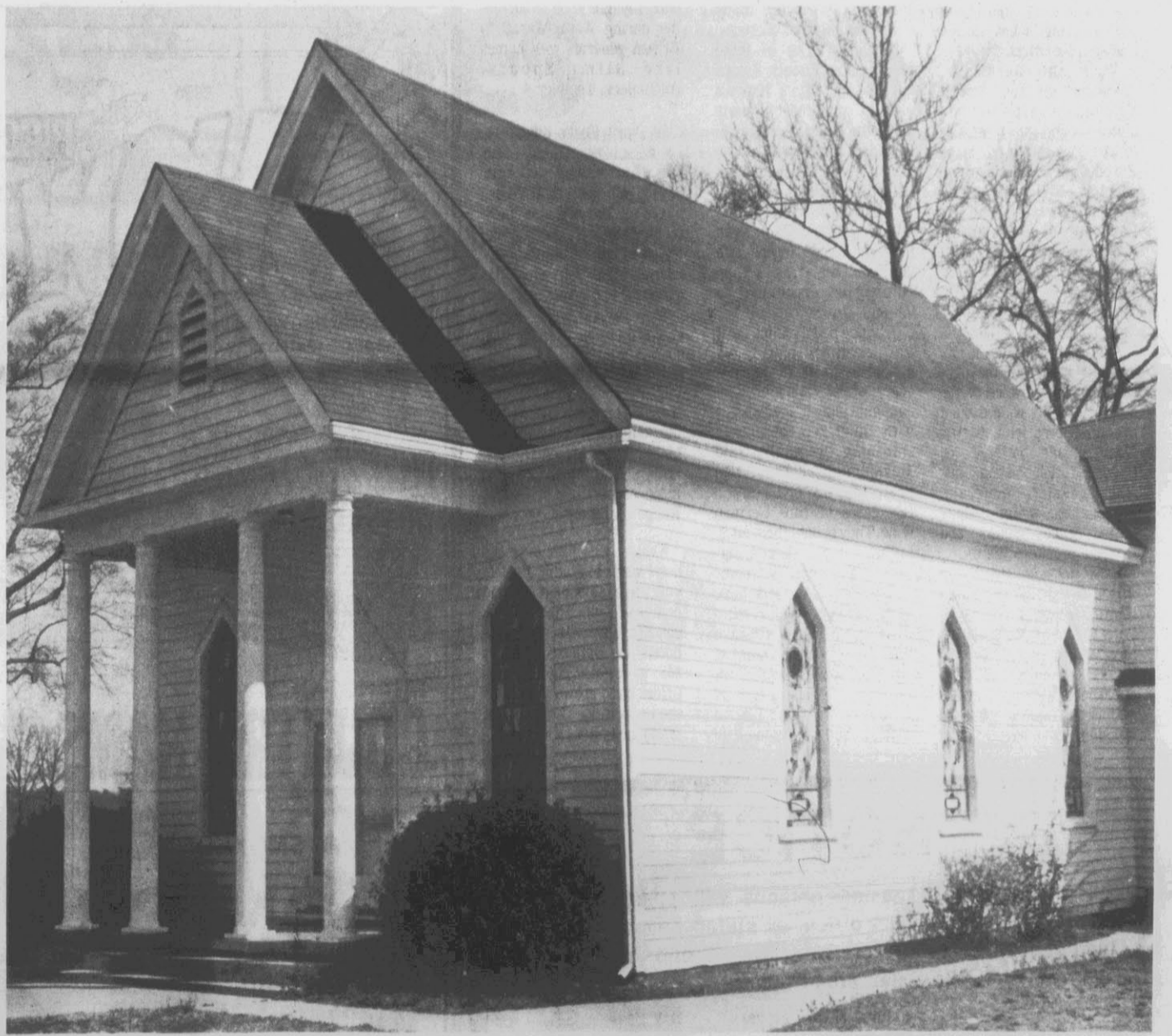
Pactolus Baptist Church is a good example of an old-style country church.
