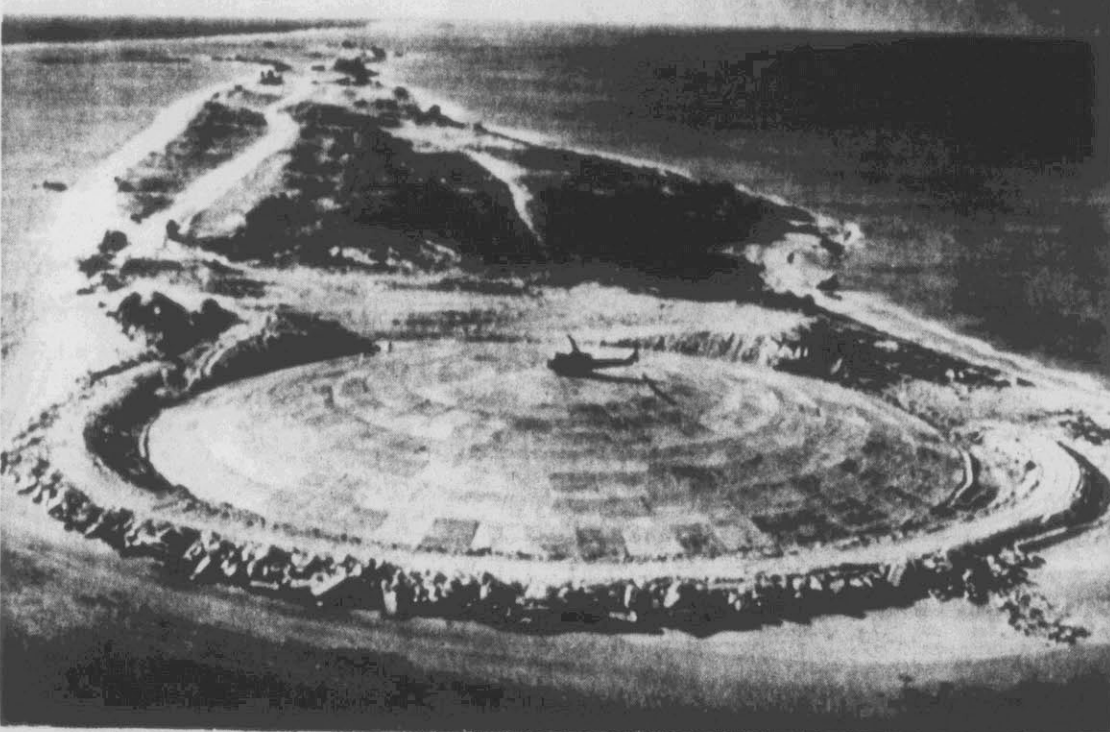
NUCLEAR TOMB — A helicopter sits recently atop an 18-inch thick concrete dome that covers more than 100,000 cubic yards of radioactive soil and debris within Cactus Crater, formed by a nuclear test explosion, on an island in the Eniwetok Atoll. The
