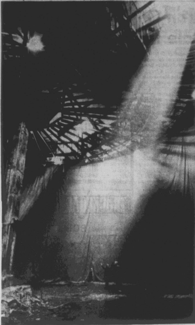
LIGHT FOR THE PAST — Shafts of sunlight pierce the dust of the restoration scene in Atlanta's Cyclorama while the building is renovated. The seven-ton painting has been
