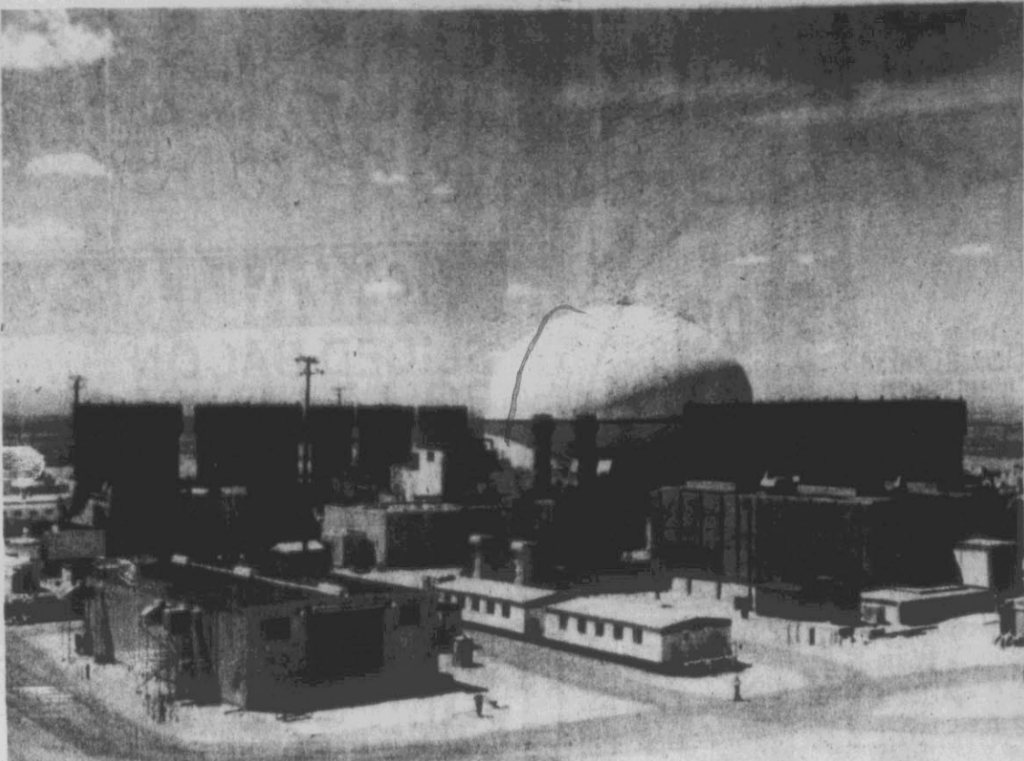
TEST BREEDER REACTOR — The Fast Flux Test Facility on the Hanford Atomic Reservation, recently achieved initial "criticality"— meaning the reactor's first chain reaction occurred deep within its
