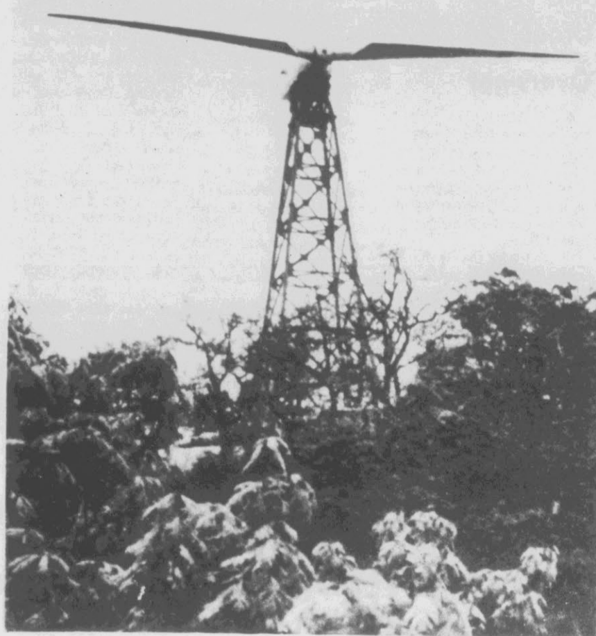
A WHITE ELEPHANT? — This is the world's largest electricity-generating windmill, sitting atop Howard's Knob in Boone, N.C. after it was dedicated July, 1979 at a cost of $3.5 million. The twin-bladed wind machine does
