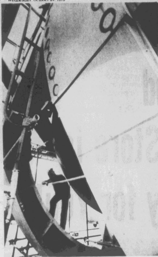
CRITICAL EYE — This steam generator going into the Waterford 3 Nuclear Station of Louisiana Power and Light at Taft, La. is getting a critical once-over from Mary Alexander Folsom. Mrs. Folsom, the only woman of 900 Authorized Nuclear Inspectors in the country, checks that the generator complies with standards and codes of the Nuclear Regulatory Commission and the American Society of Mechanical Engineers. (AP Laserphoto)
