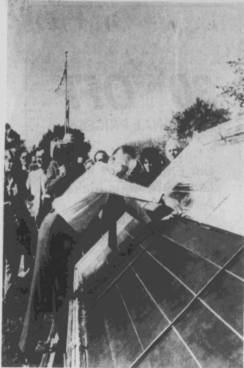
PORTABLE FARM SOLAR HEATER — Department of Agriculture Secretary Bob Bergland tries his hand at assembling a portable farm solar heating unit outside the Agriculture Department in Washington. The
