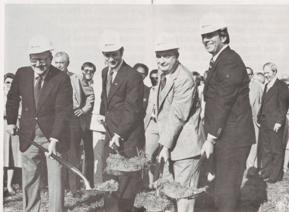
Dean William E. Laupus, Gov. James B. Hunt Jr., Chancellor Emeritus Leo W. Jenkins and Chancellor Thomas B. Brewer at the groundbreaking ceremony for the medical science building
