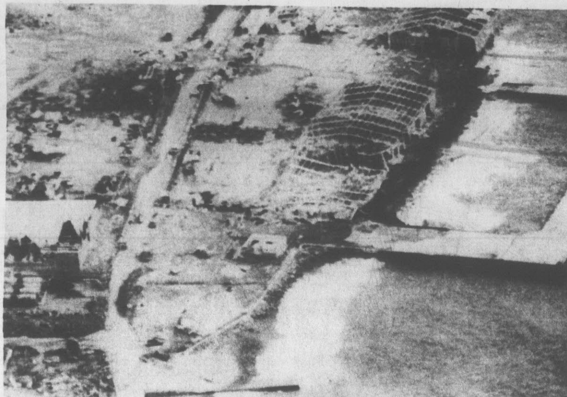
HURRICANE'S WAKE — Hurricane David completely demolished the banana crop warehouse at the new deep water harbor at Roseau, Dominica, when it struck at the island on Wednesday, leaving an estimated 26 dead and some 60,000 homeless. (AP Laserphoto)
