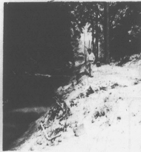
Construction work along streams is conducted from one side only. Trees on the undisturbed side provide shade needed by fish.
