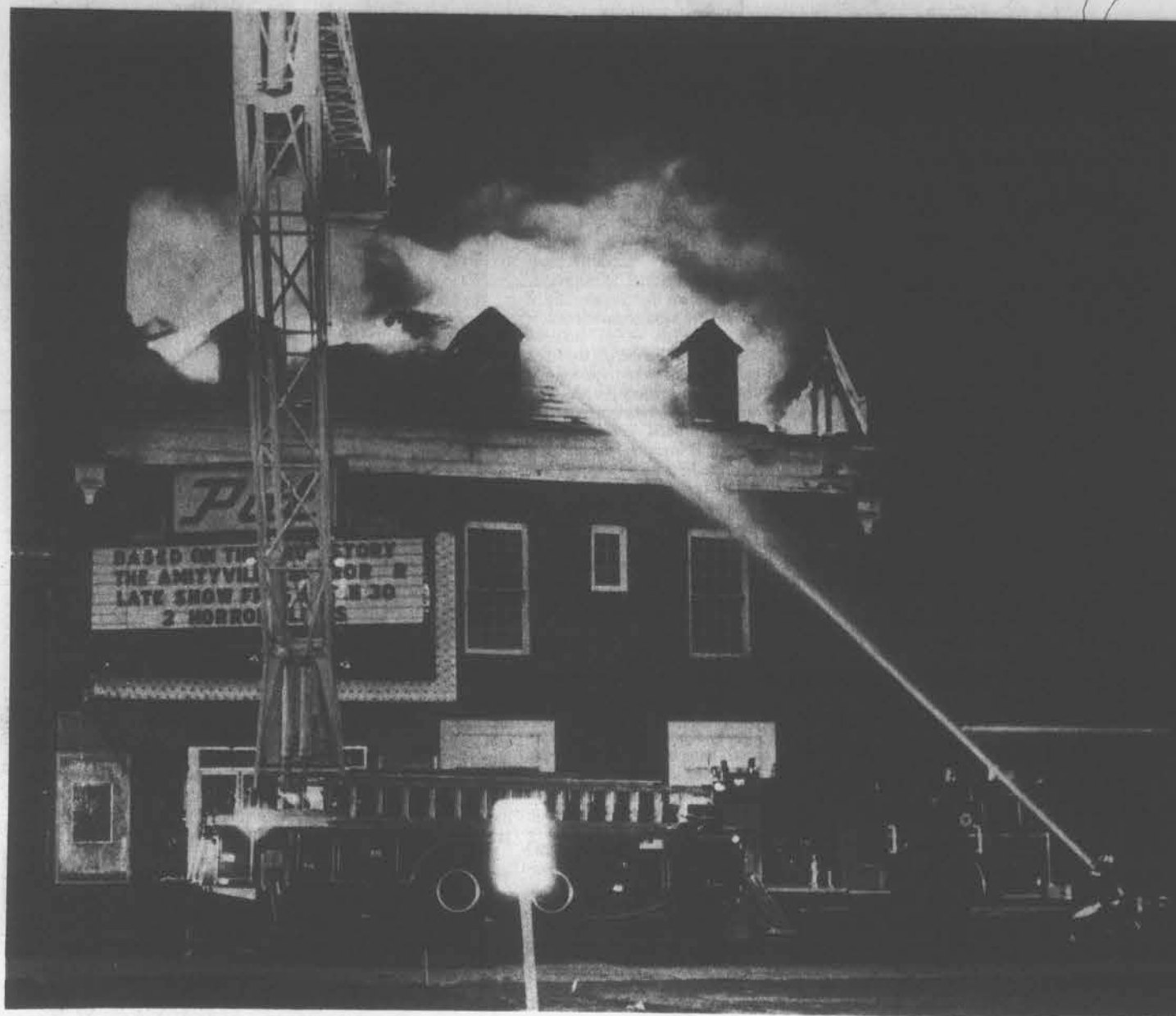
THEATER BURNS — The Greenville Fire Department snorkel unit operates above the burning Pitt Theater building. The flames broke through the roof
