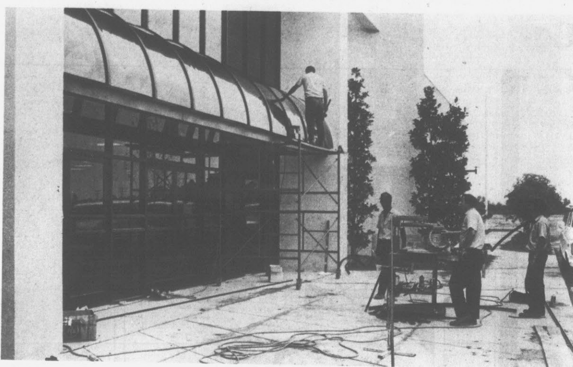
GLASS PANELS — Belk's entrance is comprised of many glass circular panels. Workmen put finishing
