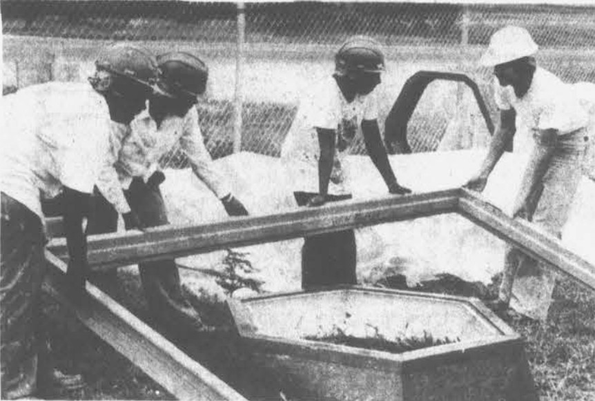
STACKING BUILDING MATERIAL . . . Three female members of the YACC — left to right, Myrtle Barnes, Diane Tyson, and Sandra Hartley, give crew supervisor Gene Wooten a hand in tidying up building material which will be used to construct a reception center.
