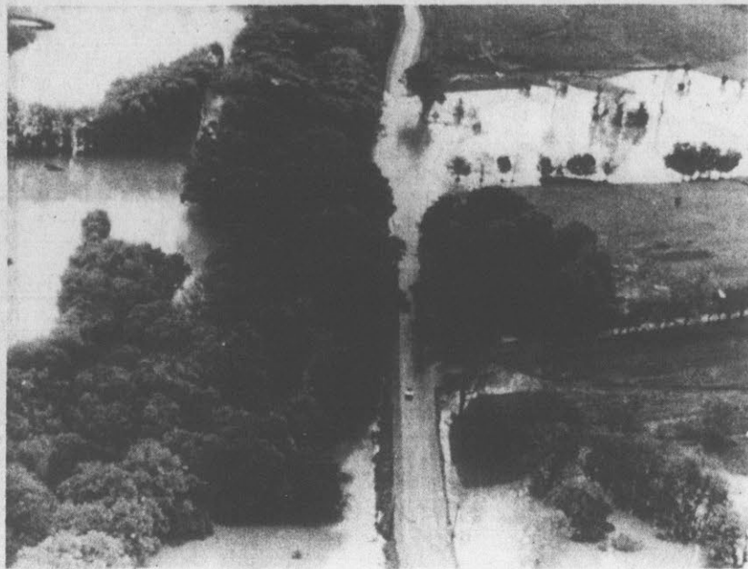
ROAD BLOCK — A thunderstorm which dumped more than seven inches of rain on middle Tennessee caused this rural road blockage near here Friday. Over 100 persons had to be
