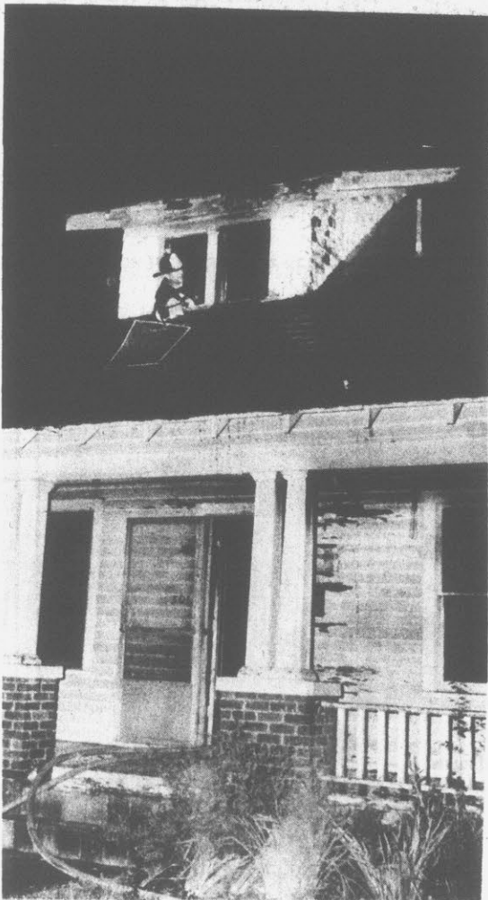
Fire Damages House
