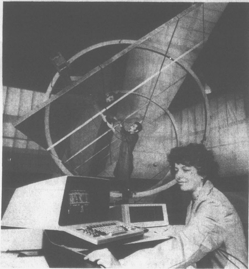
SUN-TRACKER — Westinghouse Electric Corp. employees put the finishing touches on a demonstration heliostat, which will track the sun across the sky and aim reflected solar rays
