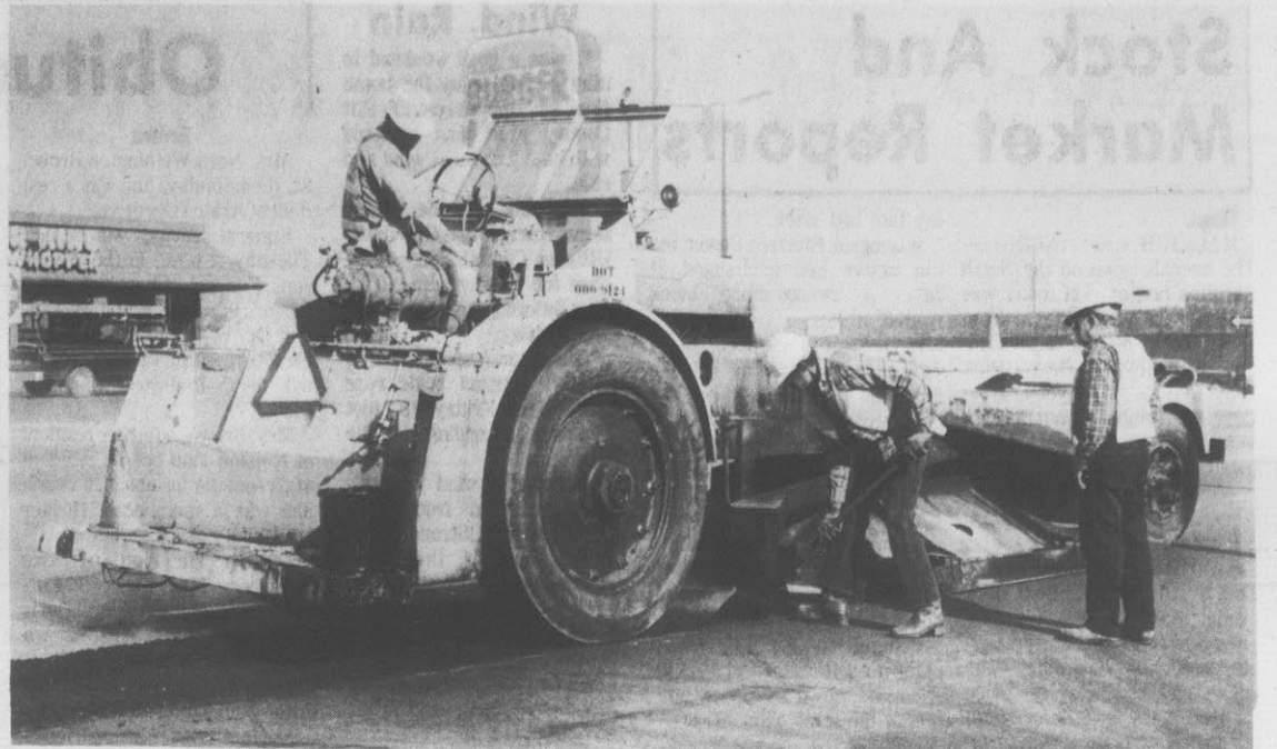
SMOOTHING OUT THE BUMPS — State Department of Transportation crews have been busy during recent days smoothing out pavement bumps on various sections of Greenville Boulevard. Workers here use the department's heater-planer machine, which directs intense heat to the pavement and planes
