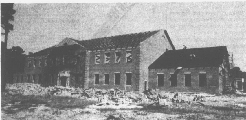
MARCH 1979... completion date is planned for the 26,000 square foot building shown here under construction. The new building will
