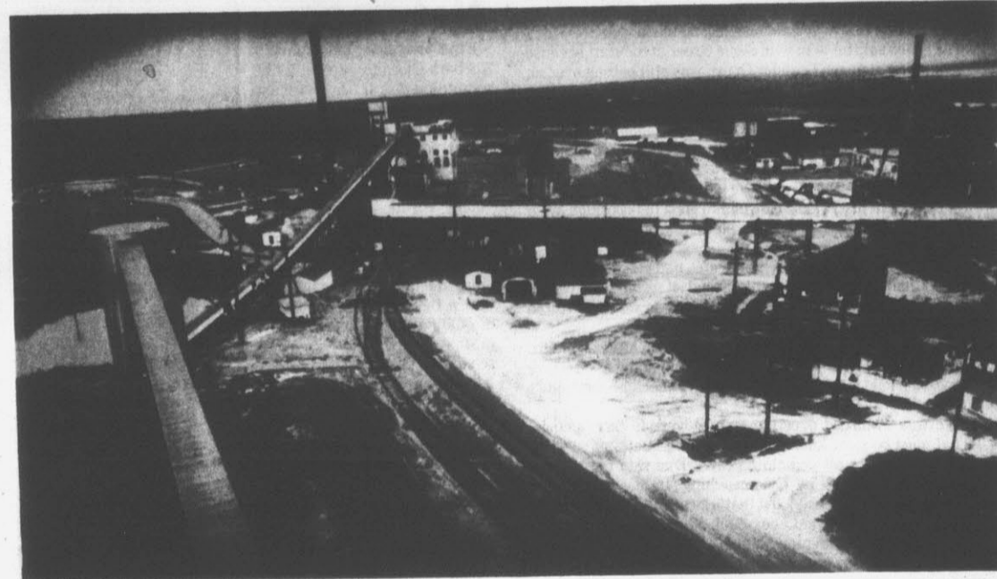
TO BE OIL STORAGE FACILITY — The Morton Salt Co. mine at Weeks Island will soon become an underground storage facility for 76 million barrels of oil. The petroleum is being stockpiled to be used if needed during a crisis similar to the Arab oil embargo. (AP Laserphoto)
