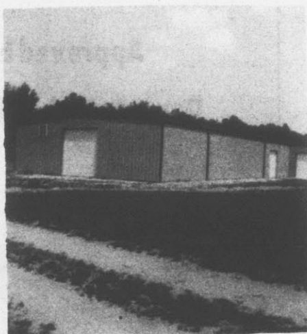
Exhibit Building In Final Stages of Construction....
