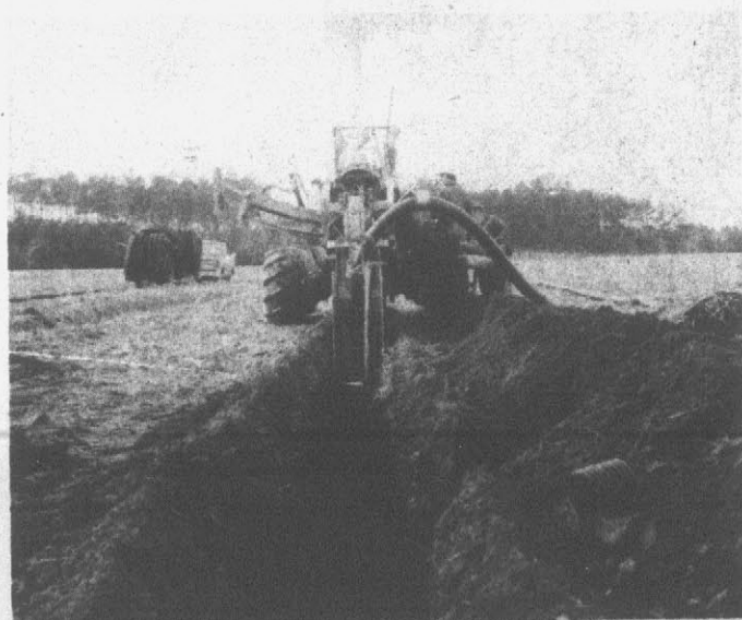
Approximately 160,000 feet of SUBSURFACE DRAINS were installed by District Cooperators to improve their poorly drained soils.
