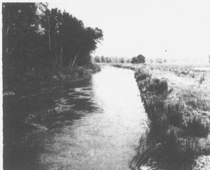
Grindle Creek Watershed Channel - Completed Area residents in Chicod, Little Contentnea, and Swift Creek Watersheds will have similar completed Channels which will help protect the farm lands from flooding and will also improve drainage.
