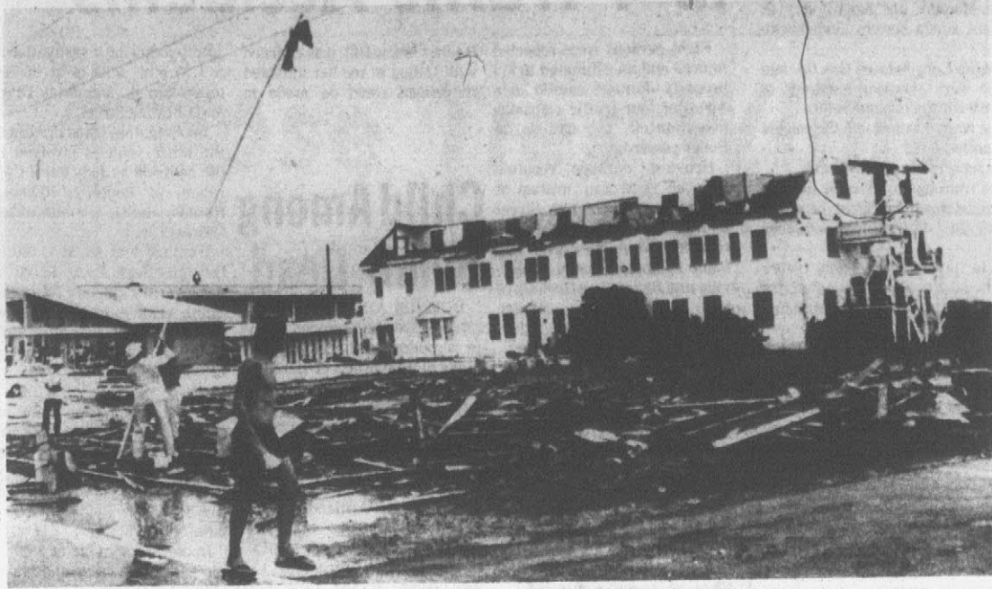
WATERSPOUT DAMAGE —The Wilbur Wright Motel in Kill Devil Hills stands derelict with debris surrounding after a massive waterspout rose from
