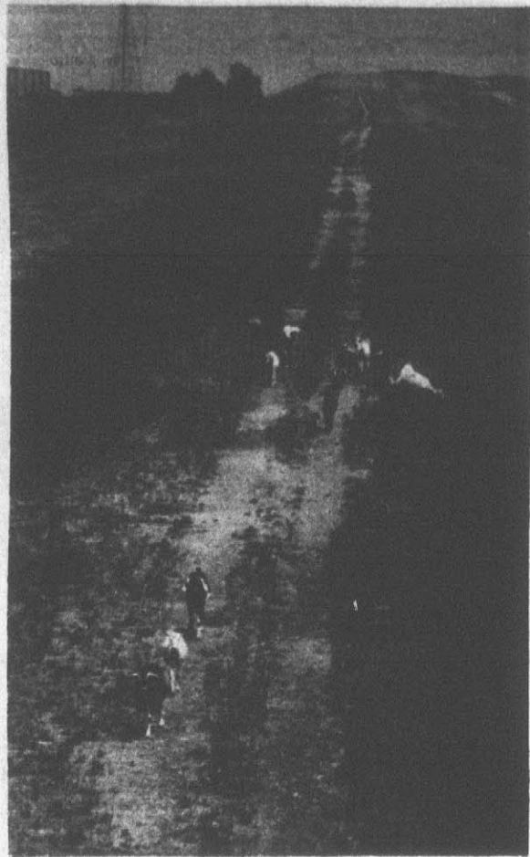
$9 MILLION GOAT PATH — Goats stroll on part of the new Route 23 that cost some $9 million to construct some 4.9 miles of super highway. When the Pennsylvania Department of Transportation ran out of money to finish the bypass from Lancaster, Pa., to New Holland, eight inches of dirt was poured onto the four-lane road and seeded. Now the goats have a good place to walk. (AP Laserphoto)
