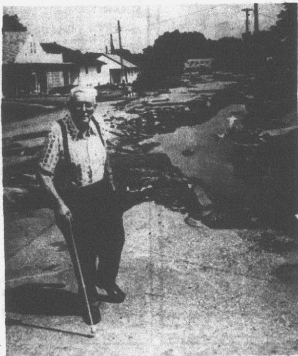
NEIGHBORHOOD WRECKED — A.L. Blackburn, 83, built many of the houses on this block where he lives. But floods, which hit Rochester, Minn. early Thursday, left a path of destruction and five deaths. Residents now face the task of rebuilding. (AP Laserphoto)
