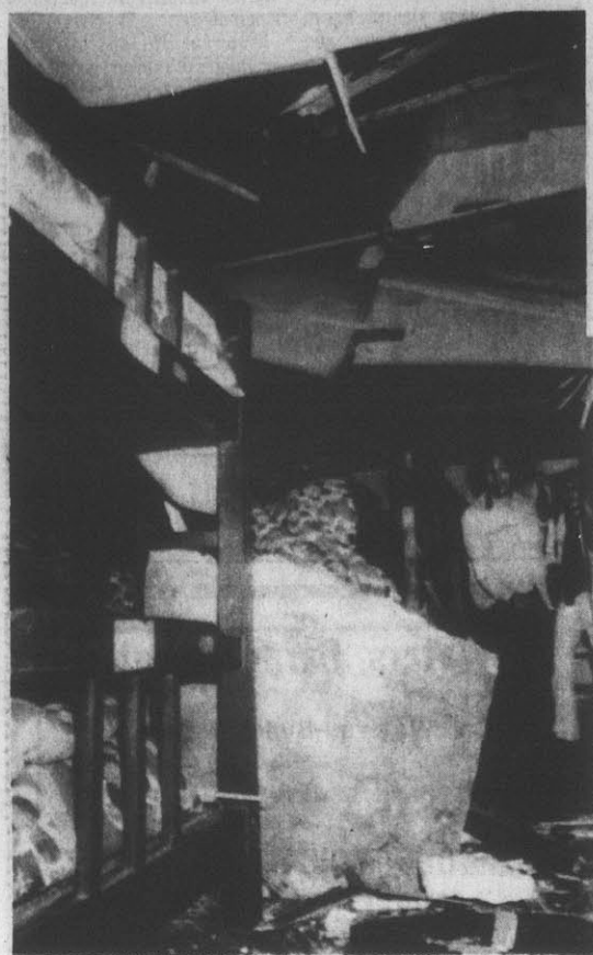
QUAKE DAMAGE — A piece of a cement chimney pierced through the ceiling of a dormitory house in Tokyo Monday, injuring two persons, following a strong, rolling earthquake. (AP Laserphoto)
