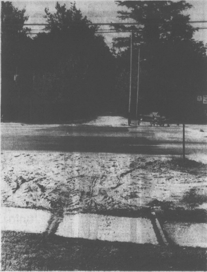
NO TRACKS ... The spur track which for years has served East Carolina University's main campus has been removed from its roadbed between Tenth and 14th Streets. Short sections
