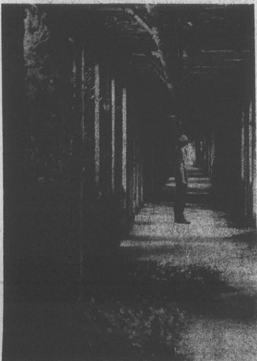
Weeds accumulate inside Ellis's decaying walls.
