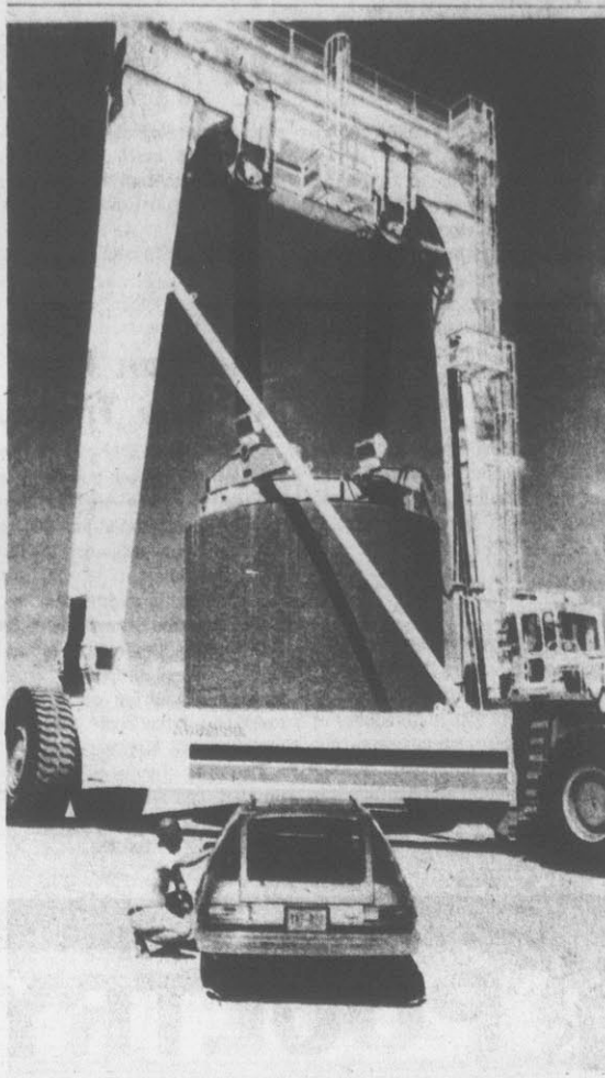
TALL TALE — A 78-foot-tall "Liftmobile", or mobile lifting device, dwarfs an automobile in foreground recently as it hoists a 115-ton section of concrete pipe, in the Arizona desert. The device is being used in construction of a water line across the state. The Liftmobile rides on 12-foot-high tires, developed specially for earthmoving equipment. (AP Laserphoto)
