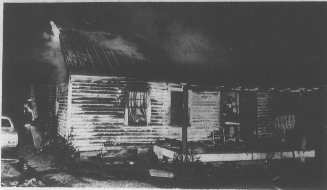
HEAVY DAMAGE. ... was done to the home of Eleanor Dupree on the Old River Road near Belvoir last night. The Belvoir Fire Department was assisted by the Falkland and Staton House
