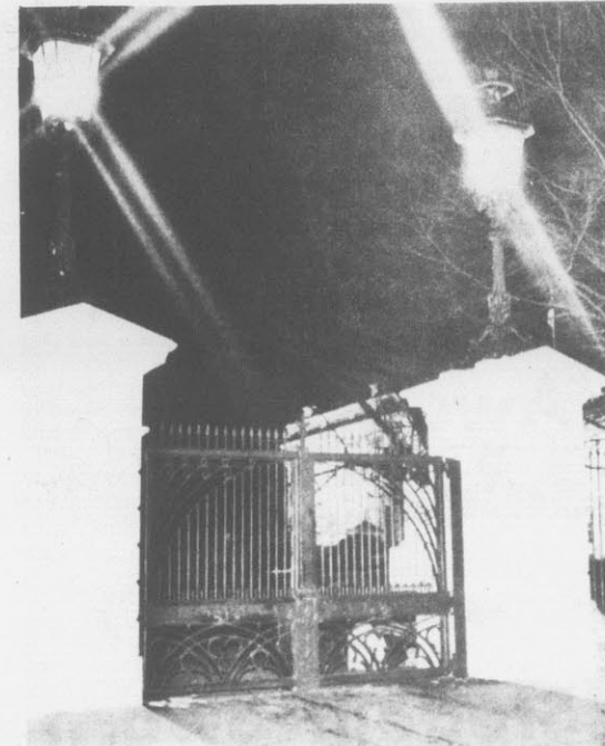
LITTLE DAMAGE — A few pieces of metal on the ground and some missing paint on the gate are the only indications of damage at the northeast gate of the White House last night after a man rammed the gate with his automobile. The gate did not give way and a man was taken into custody shortly after the incident. (AP Laserphoto)
