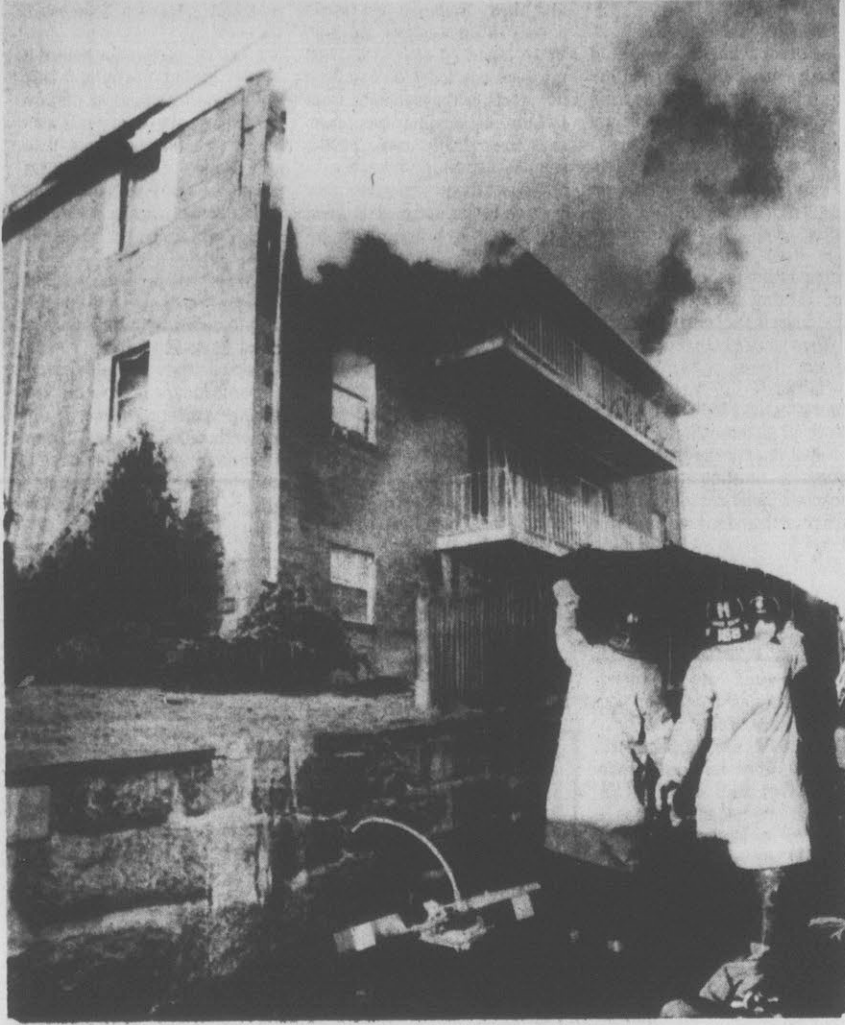
COPTER HITS APARTMENT — Parts of a radio station traffic helicopter lie on the ground beside a burning apartment building in Quincy, Mass. The craft, from Boston's WEEI, crashed into the roof of the building. (AP Laserphoto)
