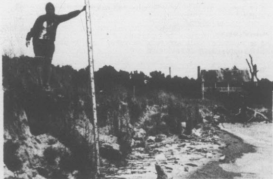
EROSION... Along the shorelines of North Carolina, erosion is a serious problem. The scene shown here is typical of the damage that can be caused by erosion. Dr. Stanley Riggs will show slides and speak on this subject at Monday night's meeting of the Sierra Club, to which the public is invited.
