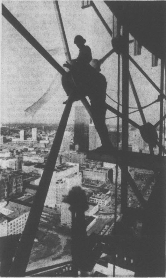
WORK ON THE DOME — Workers connect struts on the geodesic dome surrounding the 562-foot Reunion Tower in Dallas, Texas. The globe, 118 feet in diameter, surrounds the tower's three levels, a revolving cocktail lounge, revolving restaurant and an observation deck. The tower is scheduled for completion this month and will become a Dallas landmark. The shadow of the tower is shown on the city below. (AP Laserphoto)
