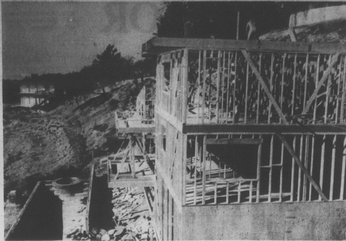
REBUILDING BURNED HOMES —A homeowner stands atop his home as it is being rebuilt amidst the blackened hills four months after the fire that burned 250 homes in the hills above Santa Bar-
