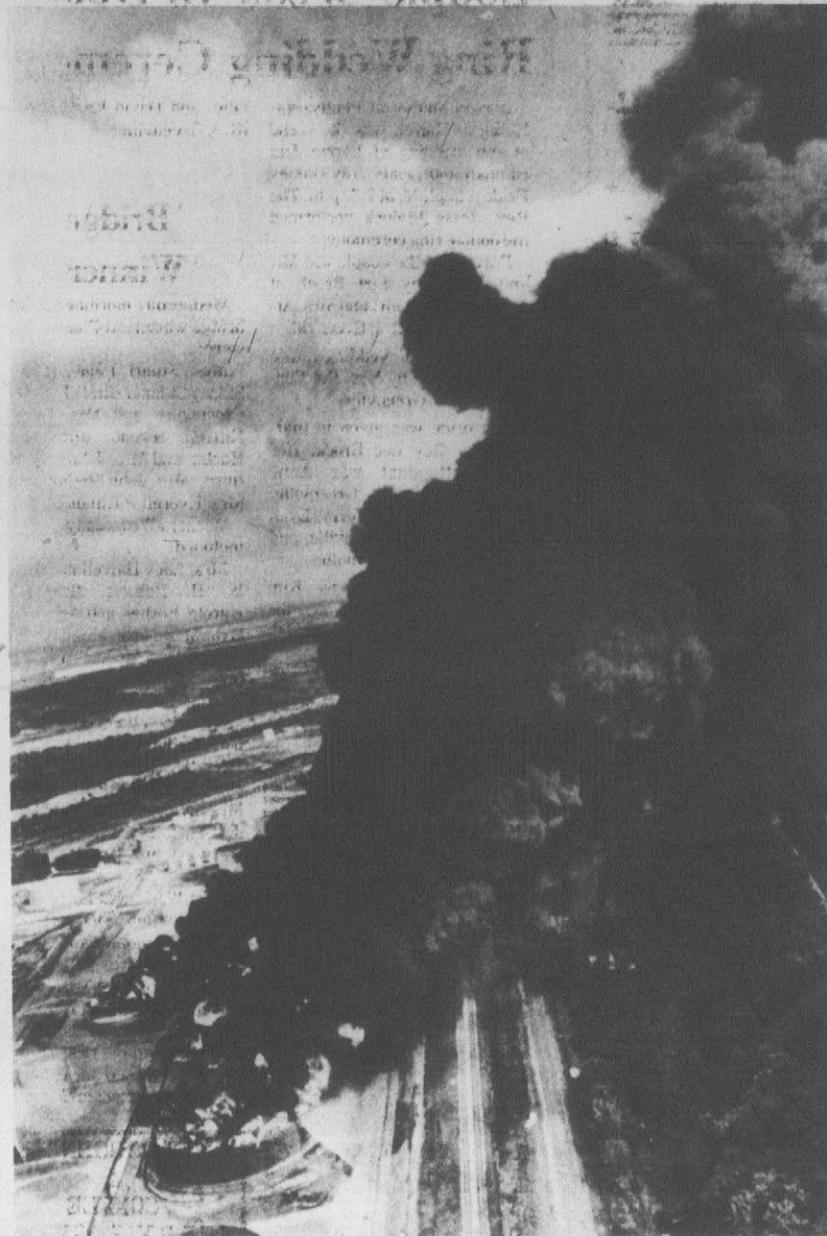
OIL STORAGE FIRE — Blazing gasoline and fuel oil storage tanks pour thick smoke high into the air at Union Oil Co. storage plant at Romeoville, Ill., southwest of Chicago, in an aerial photograph made Saturday. The fire con-
