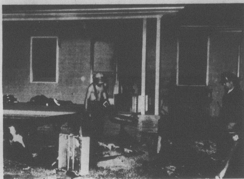
FIRE DAMAGE — Fire damaged a dwelling at 102A Holly St. early this morning. Fire officers, who said the blaze was reported at 4:32 a.m., said the fire apparently started on a couch from a cigarette and spread to other areas of the living
