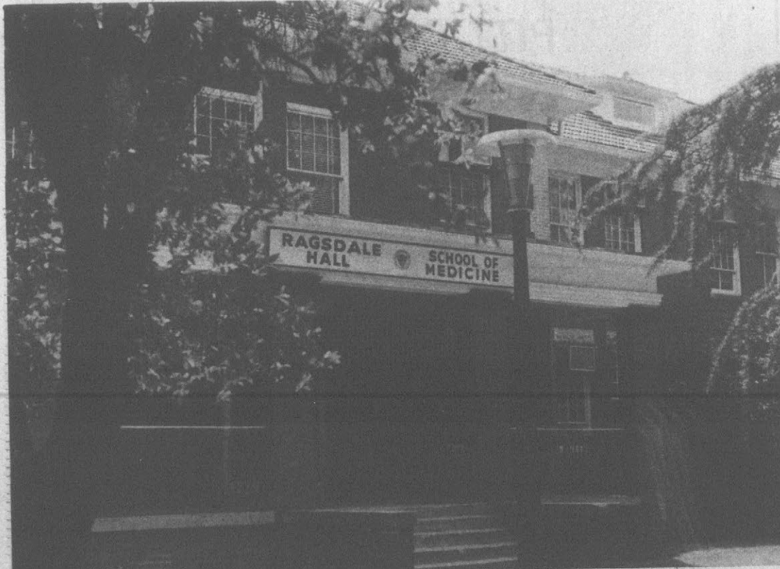
RENOVATED RAGSDALE HALL — One of the older buildings on the East Carolina University campus, Ragsdale Hall was renovated into office, classroom
