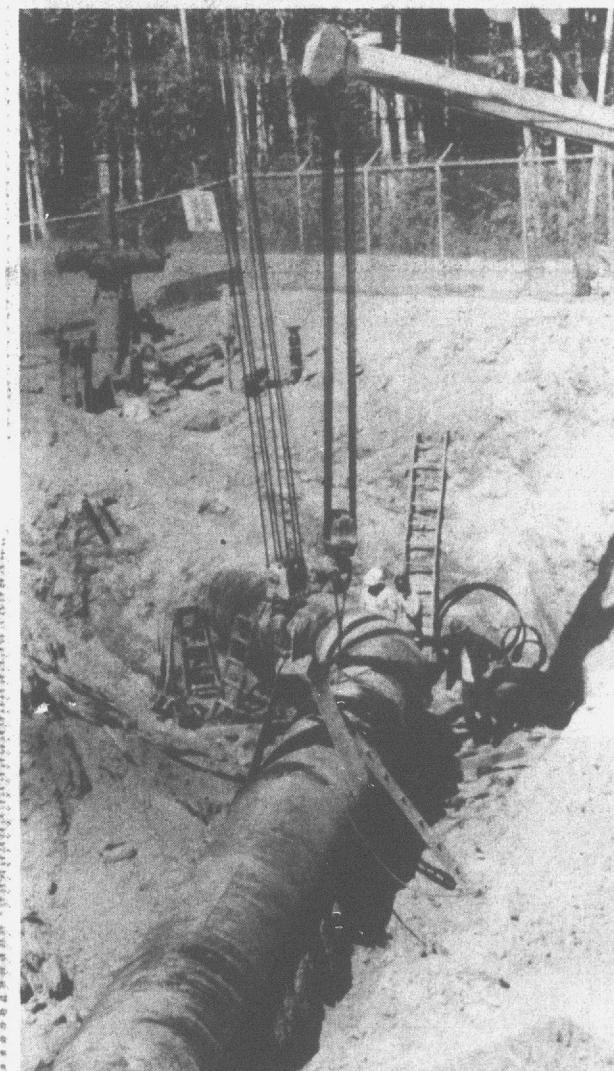
REPAIRING THE LEAK — Workmen repair a cracked elbow joint which forced a shutdown of the Trans-Alaska oil pipeline Monday evening. The crack was apparently caused by the injection of supercold liquid nitrogen instead of gaseous nitrogen into the 48-inch line from Prudhoe Bay to Valdez. (AP Wirephoto)
